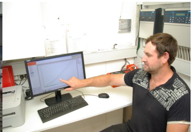
Systemet tjekkes for alarmer
